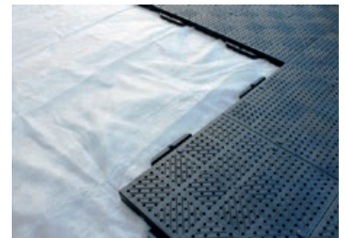
Figure 2: Laying on Geo-Tarp
