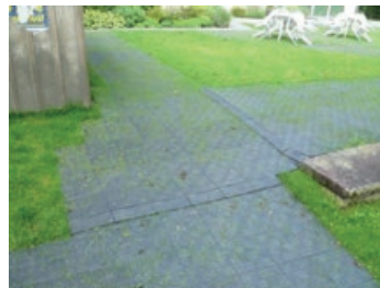
Figure 1: Laying without Geo-Tarp - the grass can grow through the tiles
